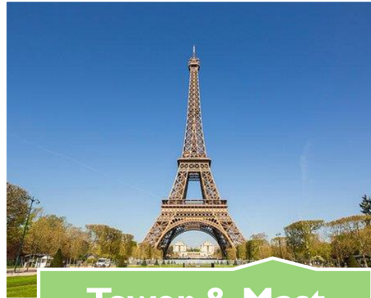
Tower & Mast structures
