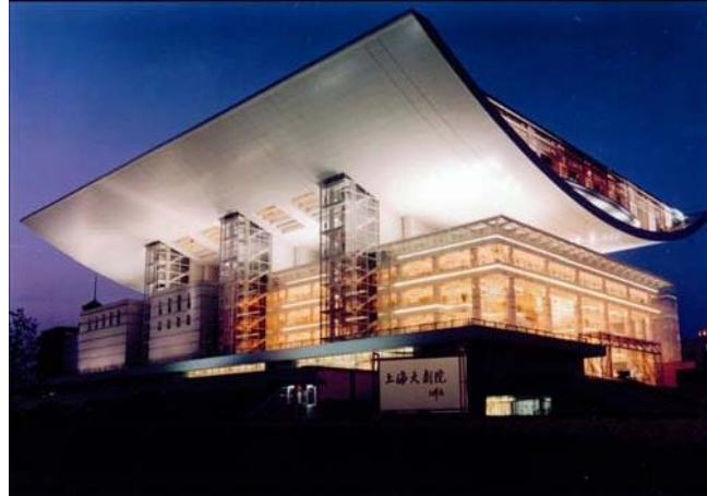
SHANGHAI GRAND THEATER Steel roof, concrete columns
