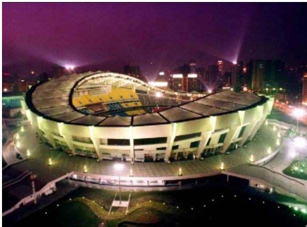
SHANGHAI STADIUM Steel roof, concrete stand
